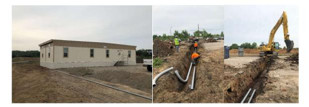
Erosion control and site demolition has been completed. This includes the removal of old water lines, gas lines, telecom, power, and sewer from the site. The building pad has been cleared and graded. Rock crushing for the drainage blanket has begun. Its installation is set to be completed in late August. Kissick continues to import fill material and is stockpiling on site.
