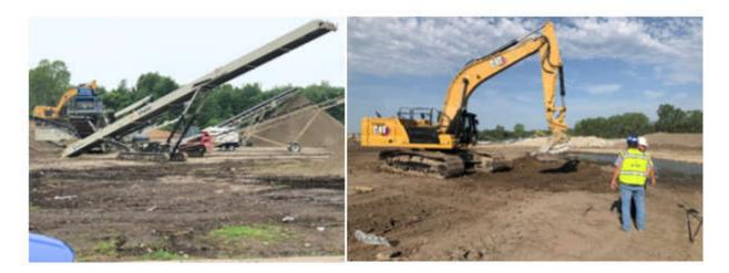
Two crusher/material classifiers are on site classifying crushed concrete, aggregate, and asphalt from stockpiles recycled from on-site demolition. Gravel and aggregate are being placed to the side of Ewing Avenue for later use. All construction activities remain on schedule.
