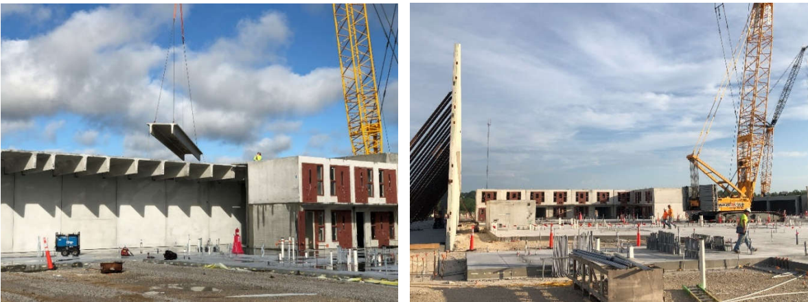
Pictured above: continued precast wall panel placement both architectural and structural.
