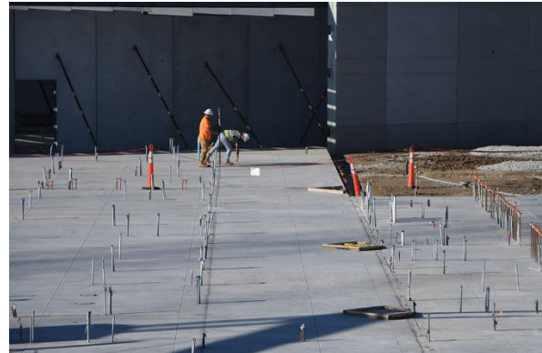
Above: Slab on grade pours and foundations are complete with all underground utilities run below.
