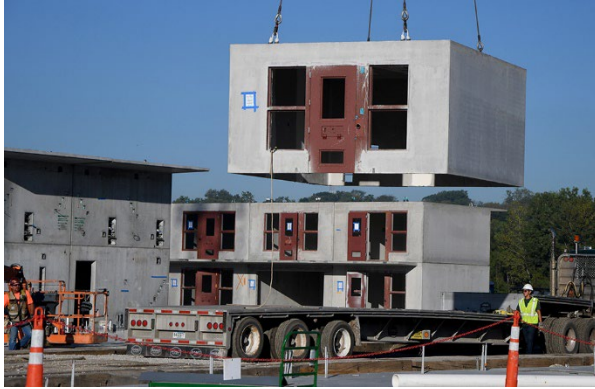
Above: All modular cell units have been delivered and installed on site.
