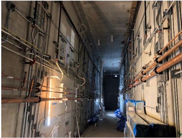
Above: Images of the rear chase behind the modular cells providing back of house access to mechanical, electrical, and plumbing systems. On the other side of the modular cells, a view of the dayrooms with roof enclosure overhead.
