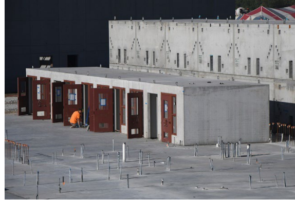
Above: All modular cell units have been delivered and installed on site.
