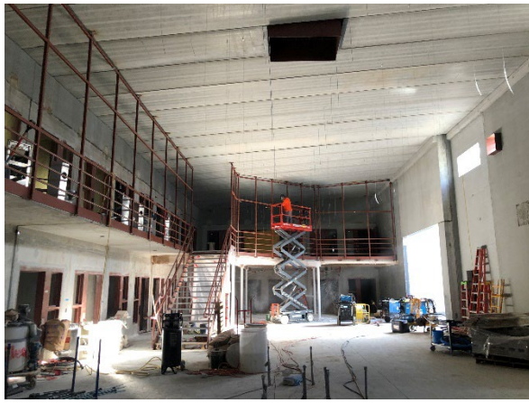
Above: Images of the rear chase behind the modular cells providing back of house access to mechanical, electrical, and plumbing systems. On the other side of the modular cells, a view of the dayrooms with roof enclosure overhead.
