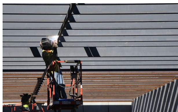
Above: Steel erection is complete at the Administrative Building at the southern facing front of the building, with decking installed and the second floor ready for a concrete slab pour.
