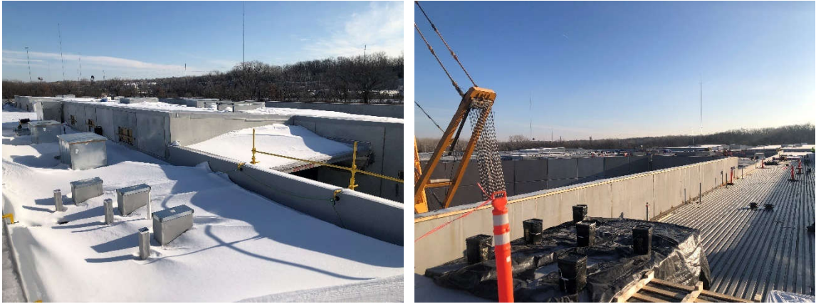
Above: Future area for the Courts prepped and ready for spray-on fireproofing.
