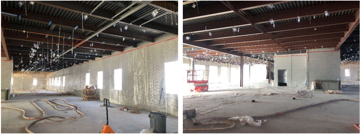
Above: Future area for the Courts prepped and ready for spray-on fireproofing.
