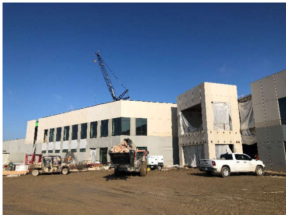
Above: Window installation on the south public facing façade of the administrative building.
