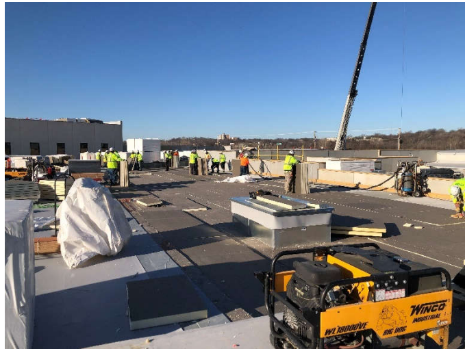
Above: Roof top equipment installation is ongoing as the last areas of roofing insulation and membrane are being installed. Roofing is scheduled to be completed this month.
