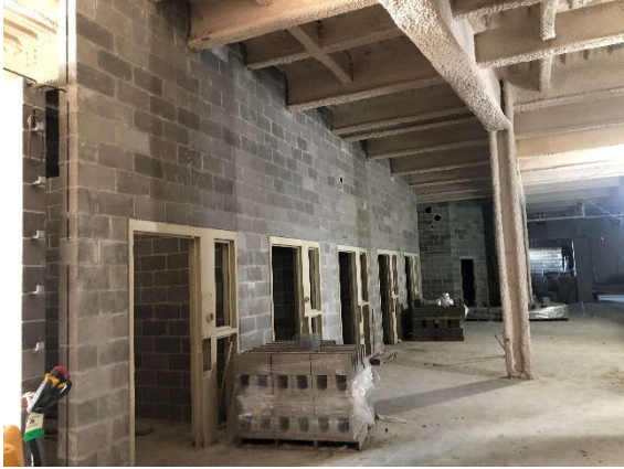
Above: Masonry partition construction continues to advance within the interior of the building.
