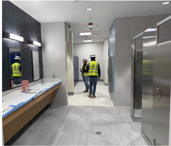
Below: Staff Locker Rooms
